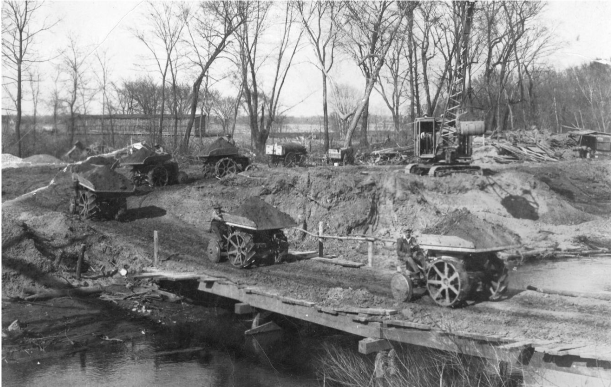
Hauling dirt on temporary bridge over English River during the drainage district project. A mobile shovel rests on the opposite riverbank. This may have been related to using excavated material from the new riverbed to refill the winding loops, or perhaps to prepare for a bridge rebuilding effort during the larger river-straightening project. From the appearance of the site, the dredge had already moved through this area and was working downstream.
